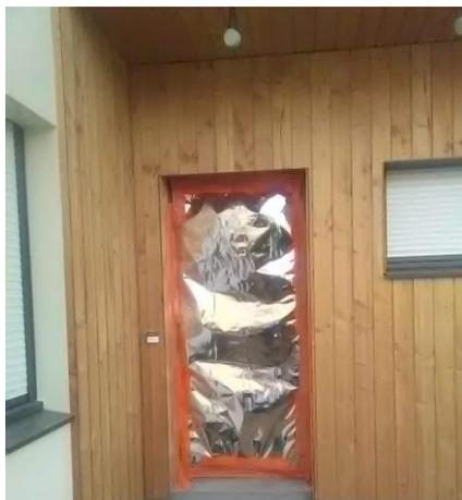
FIGURE 25: EXEMPLE D'UNE PROTECTION SOLAIRE RAPPORTEE UTILISEE SUR LE SITE DE NANTES
